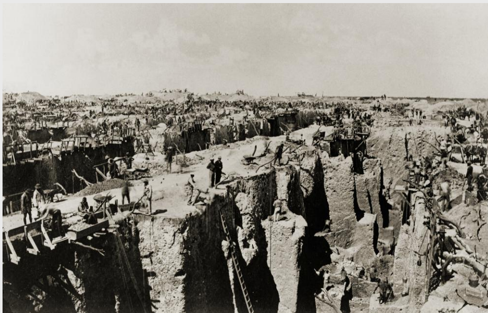
Figure B-1. Image of the haphazard mining operations at the Kimberley “Big Hole” before the consolidation of mining operations by Cecil Rhodes and Barney Barnato, and the founding of the De Beers Consolidated Mines in 1888. Each miner owned a small claim of land and sent diggings to the surface by winch and rope. They worked at different rates and left a highly irregular and dangerous surface. See also figure 1C.
